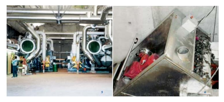
It is for this reason, that the amount of waste water required is pumped from the main channel, cleaned in a two step process (mechanically and by sedimentation) and finally is passing through the shell and tube heat exchangers of the two heat pump units. After extraction of the energy the waste water is lead back to the main channel.
